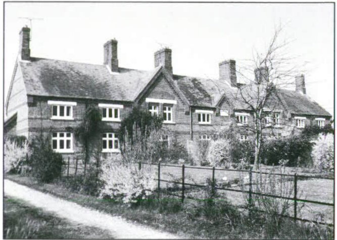
Holmwood Cottages, Main Road
