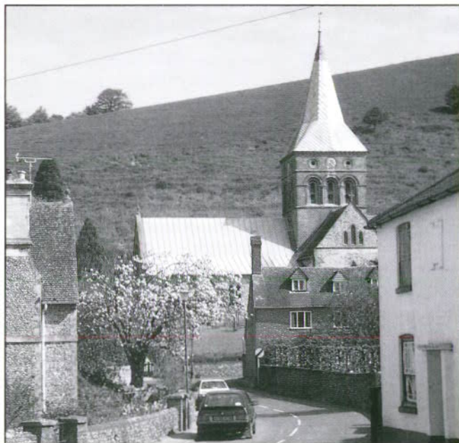
Church Street, All Saints Church is in the background.
