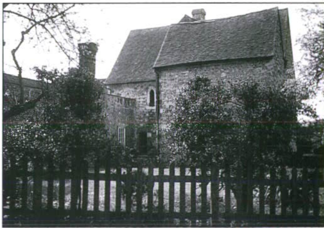
The Court-house, Church Road.
